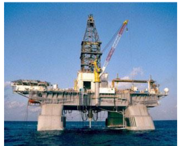
Deepwater Horizon Drilling Rig Courtesy of providingnews.com 9/11/10
